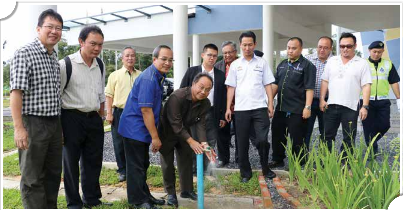
Water supply to new UiTM Campus in Mukah.
