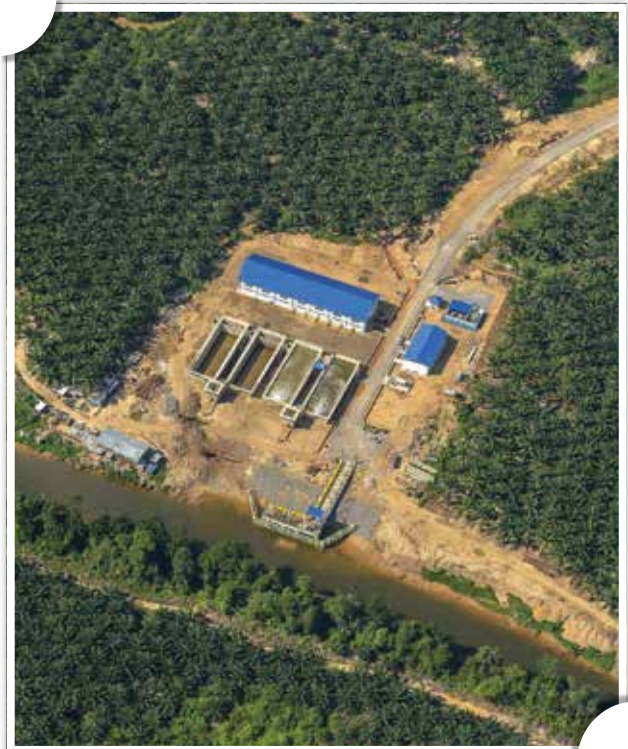
Completion of Samalaju Raw Water Intake facility.
