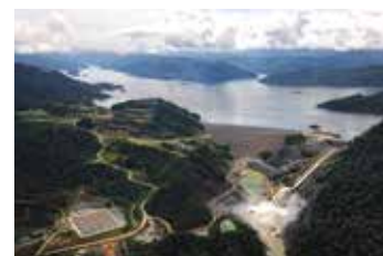
Bakun HEP begins generating electricity
