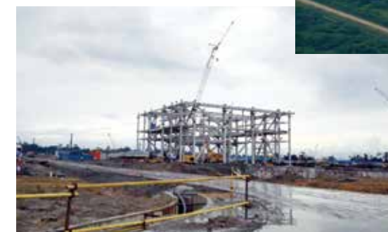
Construction of Balingian Coal Fired Power Plant begins
