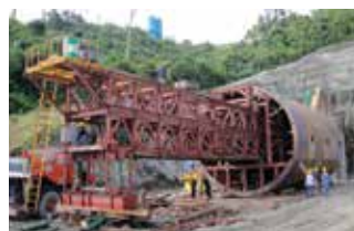
Construction of Murum Dam begins
