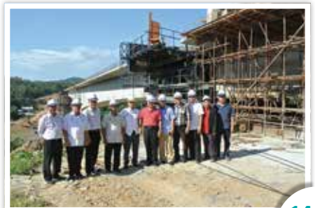
Site visit and site meeting No. 24 on Baleh Dam access road project package B (phase 1)
