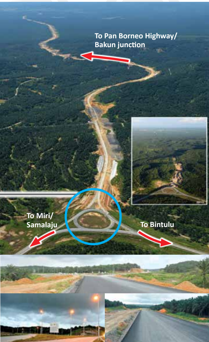
Access Road to Mile 32 Service Centre connecting to Pan Borneo Highway
