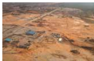
Construction of Samalaju Industrial Park begins in 2009
